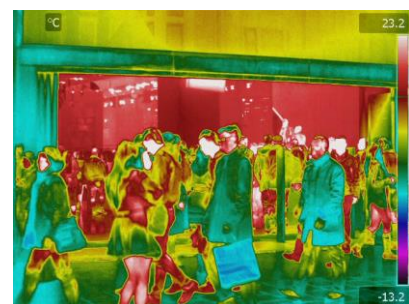
Open doors such as these can double a shop's energy use.
